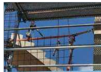
Positioning of loads
