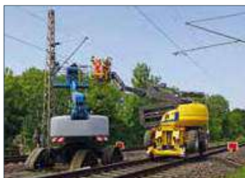
Construction of contact lines
