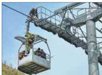
Cable car construction
