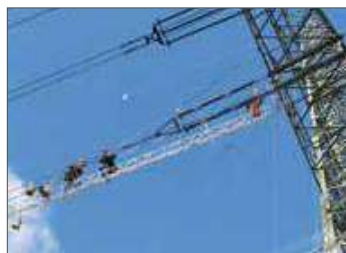
Overhead line construction
